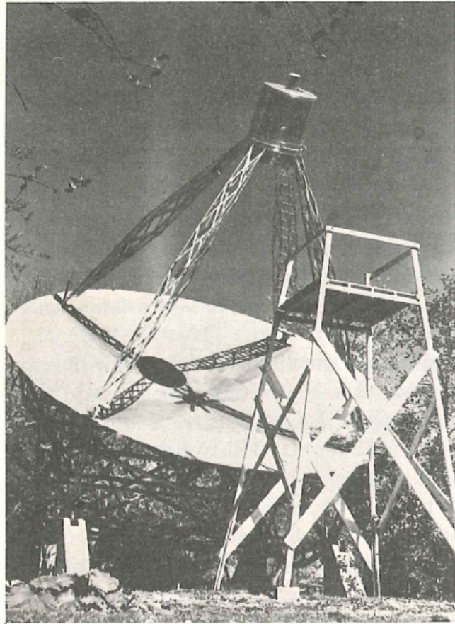
Fig. 1-5. Grote Reber's meridian-transit radio telescope. Many modern radio telescopes bear a striking resemblance to this early instrument.
