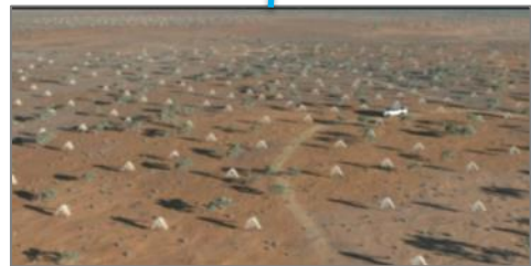
SKA1_LOW Low Frequency Aperture Array Stations 25000 antennas
