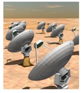
Telescope:  $36 \times 12 \text{ m}$ Beam-size: 10 arcsec Fov:  $30 \text{ deg}^2$  (FPA) Bandwidth: 300 MHzFrequency range: 700 - 1700 MHz (z < 1.38) line sensitivity (150 kms<sup>-1</sup>): 0.21 mJy/beam (12 hr) (1 $\sigma$ ) 0.73 mJy/beam (1 hr)
