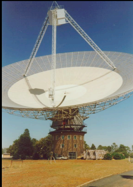
13-beam 21-cm receiver at prime focus
