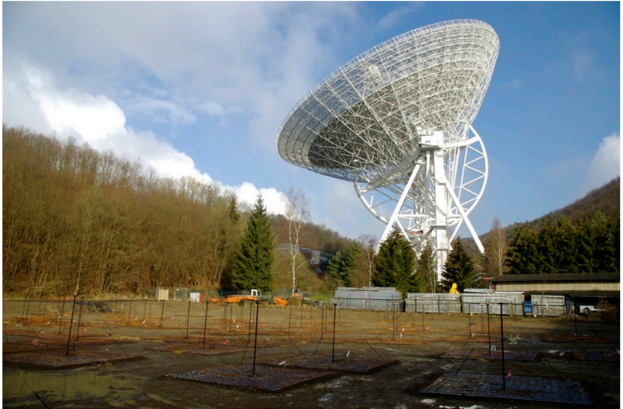
Traditional paraboloid and LOFAR aperture array telescopes side-by-side at Effelsberg, Germany.
