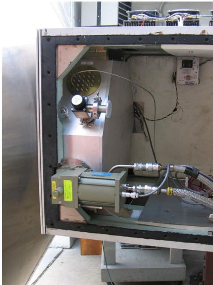
Cryostat in NRAO Front-end Box
