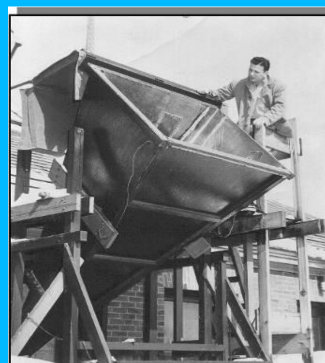
Figure 5. How Ewen expected to detect the hydrogen line. IEEE Antennas and Propagation Magazine , Vol. 41, No. 1, February 1999
