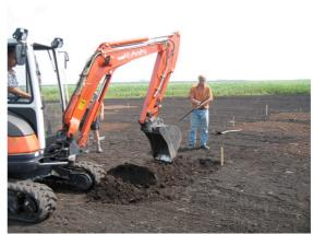
After all the positions were measured (by a geodetic company) and marked with a small wooden stick. A small crane created a trench for the 2 coax cables for the antenna.
