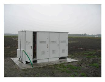
The cabinet consists of 4 compartments. The first three are used for the receiver units and the digital processing. The fourth compartment is for control, power connections, rubidium clock, local control unit etc.
