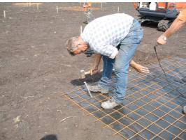
Then the 4 tension cord/springs (2 arms of the antenna have tension cords, the other two springs) are connected by 4 ground pins.
