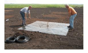
The groundplane is placed, also exactly in the wind directions. The groundplane is part of the antenna and will create a bundle towards the sky. This groundplane is "normal" construction steel (for concrete constructions) with the exception that all the crossings of the wires are welded (this is not normal for this material).
