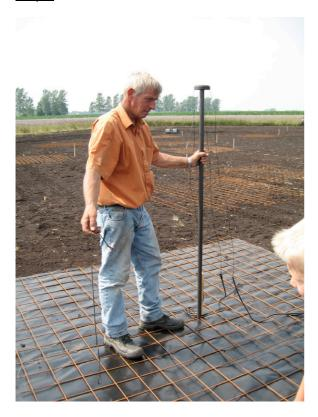
The tube has little slots in the bottom which make a perfect fit on the grid of the wire mess. The two antenna cables have a little over length at the bottom, to assemble but also disassemble the antenna easily.
