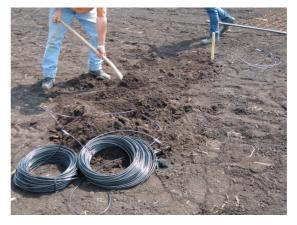
The two cables are placed and the ground is made flat again (by hand).
