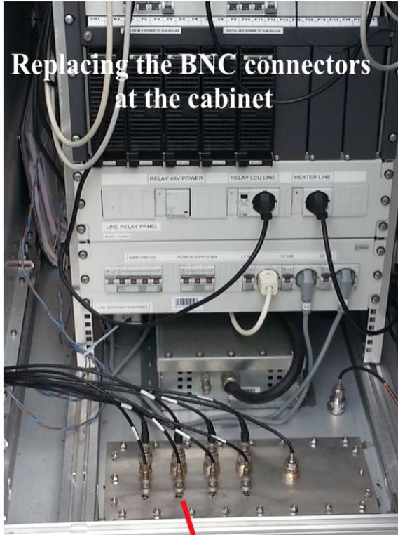
Replacing the BNC connectors
