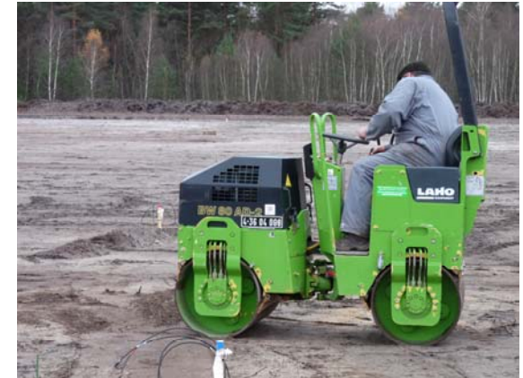
Leveling with a compactor
