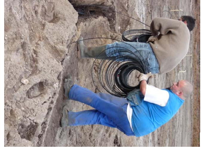
A « swimming pool » is dug for cables extra-length
