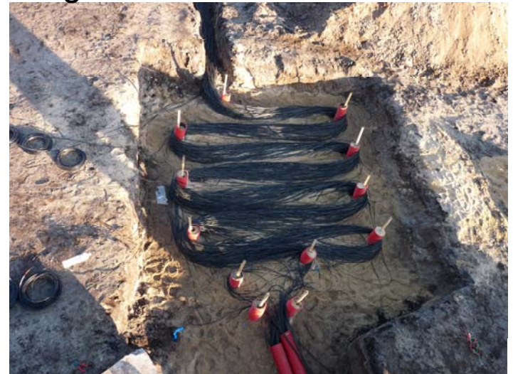
A « swimming pool » is dug for cables extra-length
