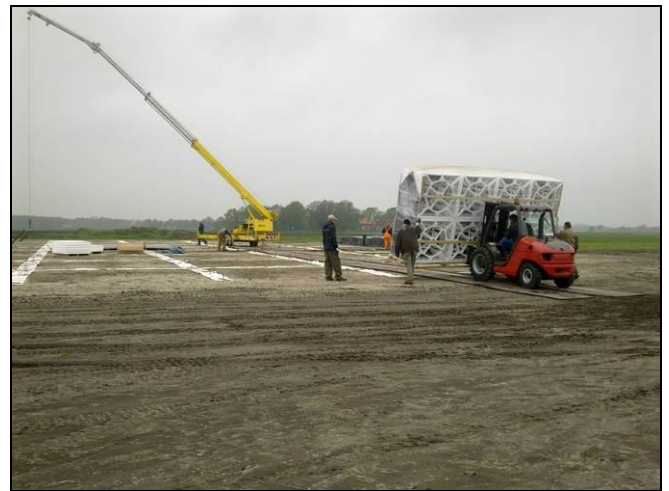
HBA-tile transport from storage trailer to installation position. (Note: POLFAR roll-out will not be executed in this manner)
