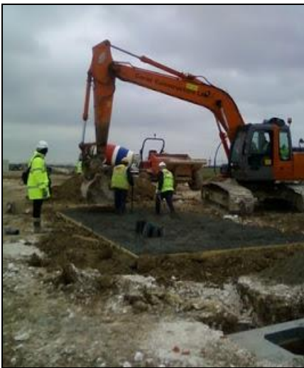
Figure 5-13, concrete base and container installation (Courtesy of UK608)
