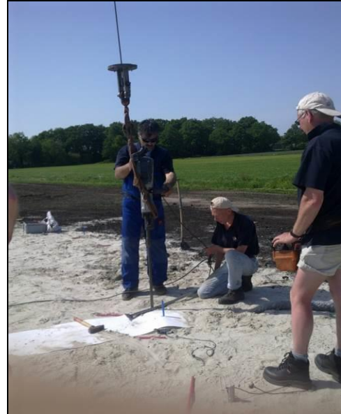
HBA-tile marking and ground anchors installation.
