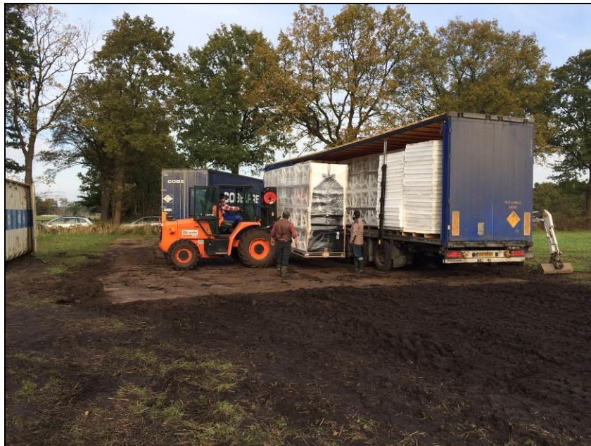
Figure 4-2 Unloading HBA tiles
