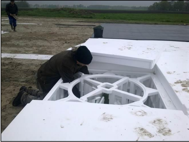
Connecting coax cables and placing top cover
