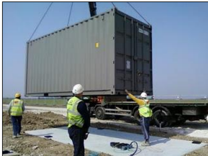
Figure 5-13, concrete base and container installation (Courtesy of UK608)
