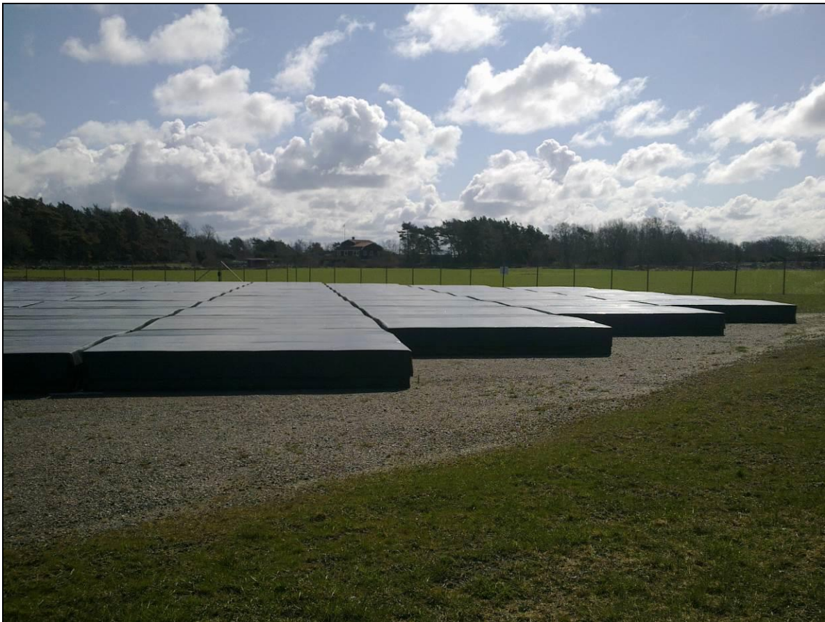
HBA final installation result (ILT SE607, Onsala)
