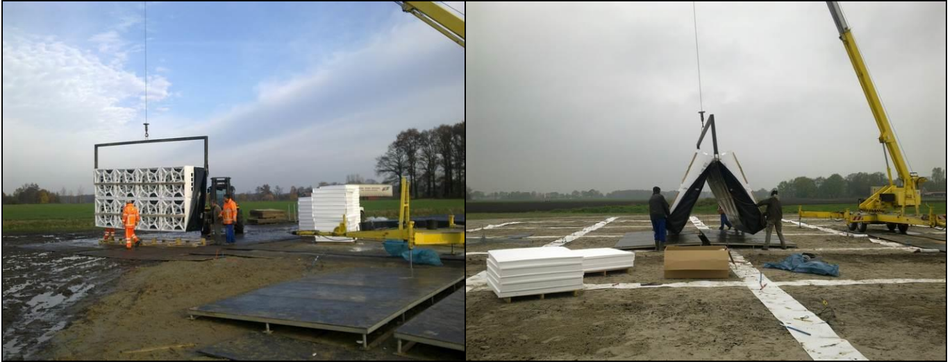
Lifting and unfolding HBA tile
