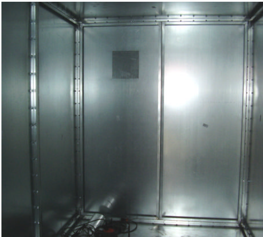
Figure: Pan-Shield type panel construction
