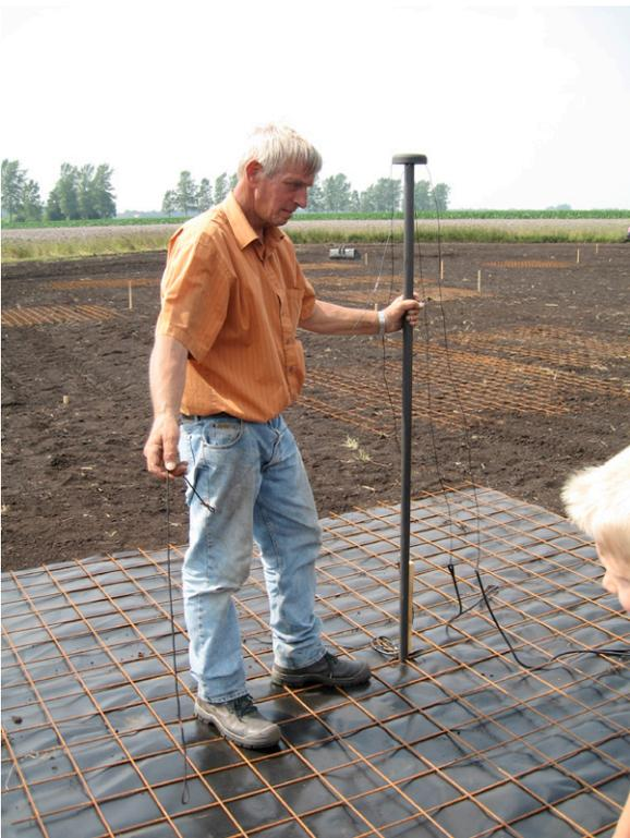
The tube has little slots in the bottom which make a perfect fit on the grid of the wire mess. The two antenna cables have a little over length at the bottom, to assemble but also disassemble the antenna easily.
