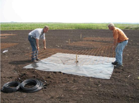
The groundplane is placed, also exactly in the wind directions. The groundplane is part of the antenna and will create a bundle towards the sky. This groundplane is “normal” construction steel (for concrete constructions) with the exception that all the crossings of the wires are welded (this is not normal for this material).
