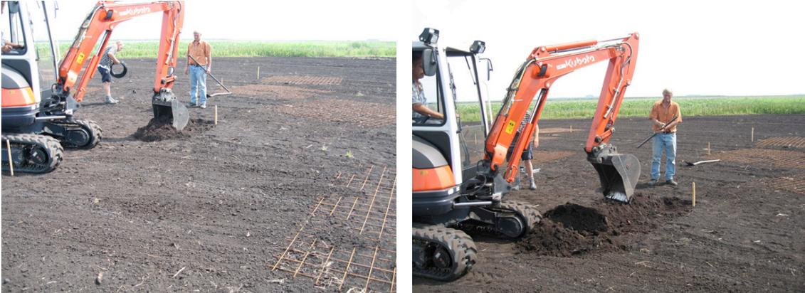
After all the positions were measured (by a geodetic company) and marked with a small wooden stick. A small crane created a trench for the 2 coax cables for the antenna.
