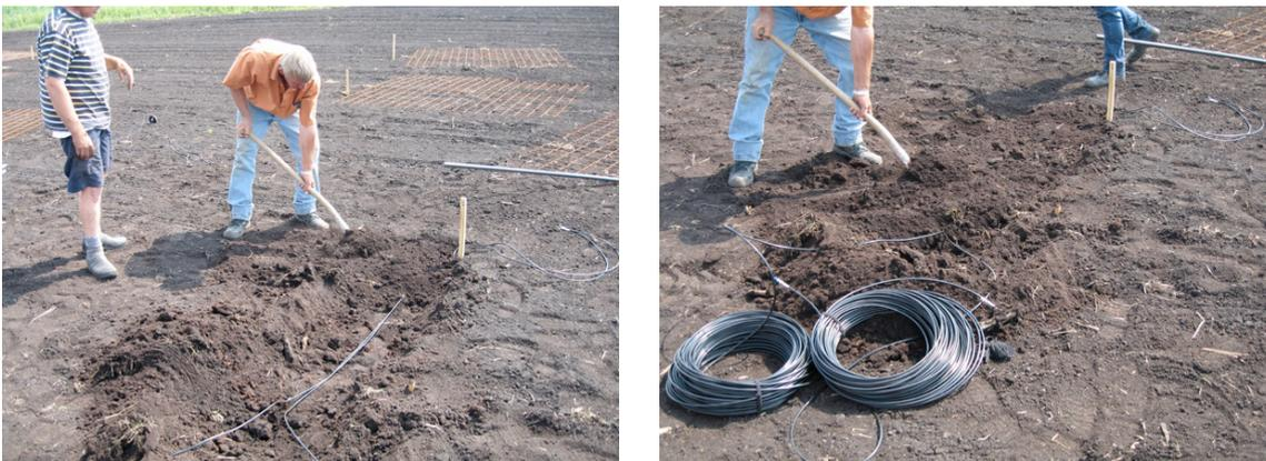
The two cables are placed and the ground is made flat again (by hand).
