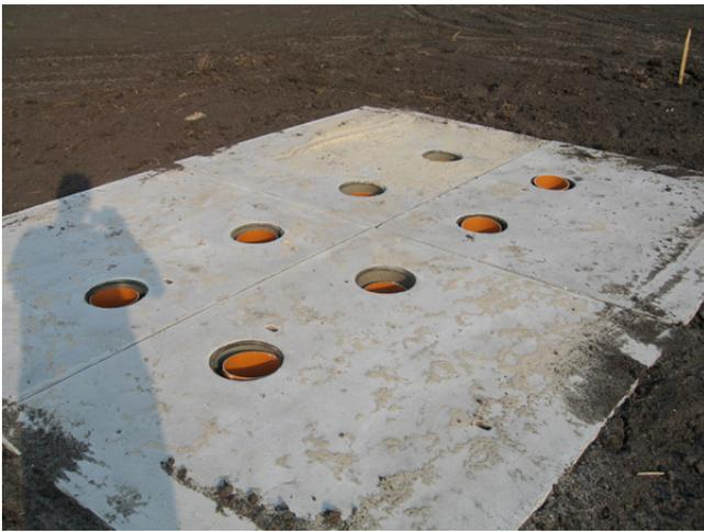
After the construction of the concrete platform the cabinet can be placed on this construction.
