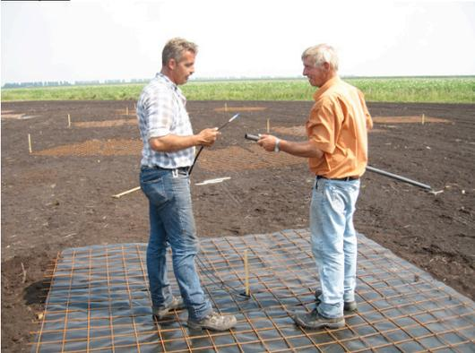
The 2 coax cables are fed into a prepared tube of exactly 1.7 meters.
