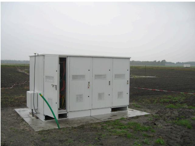
The cabinet consists of 4 compartments. The first three are used for the receiver units and the digital processing. The fourth compartment is for control, power connections, rubidium clock, local control unit etc.
