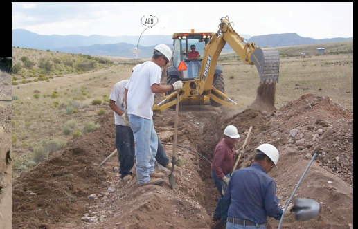
Fiber optic transmission
