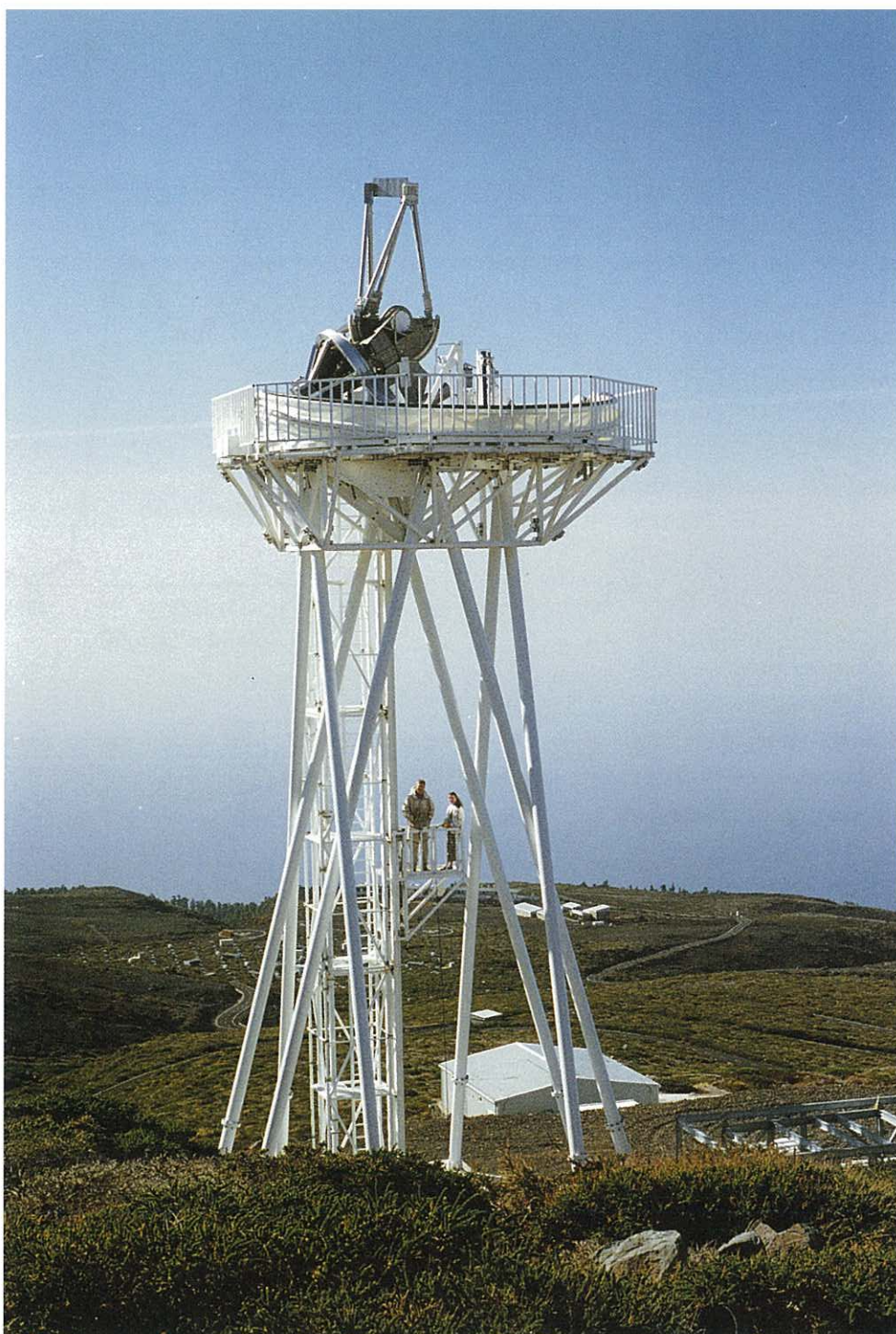
The Dutch Open Telescope installed at the Roque de los Muchachos Observatory on La Palma. The tower and telescope are designed thermally to avoid locally generated image degradation, and mechanically so they are extremely stiff and can withstand substantial winds without shaking.
