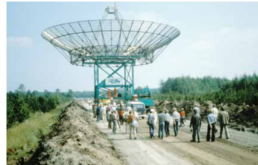
Figure 3: At the end of the 1970s 2 telescopes were added on the existing track to the original 10+2 telescopes. After they were used to get a higher sensitivity, especially for HI line observations, they were moved to a newly built track 1500 m to the East of the existing telescope. A temporary road and bridge were built to get the 50 ton telescopes to their new position. (H.J. Stiepel)
