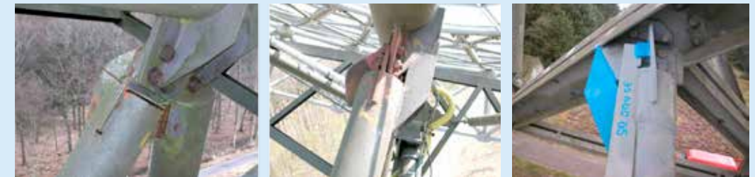
Left: RTC in 2004 connection to declination axle is completely broken. Middle: Connection to the declination axle, re-welded and reinforced on all 14 telescopes. Right: additional strengthening of the tube counterweight construction now on 12 telescopes
