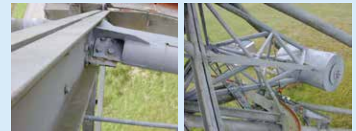
Left: A repaired tube with an additional strengthening member added. Right: Hour-angle counterweight construction, with all members doubled in steel on all 14 telescopes.
