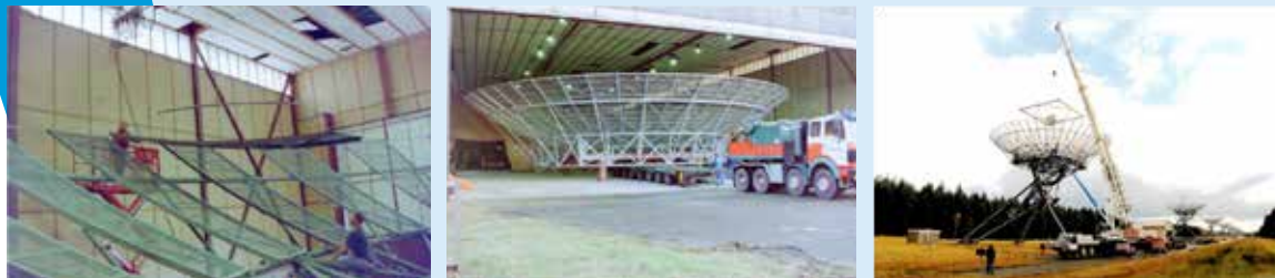
Left to right: 1994 removal of outer-panel of RT5. 1994 reflector ready for transport to RT5. 1998 November, lifting of last revised reflector on RT0
